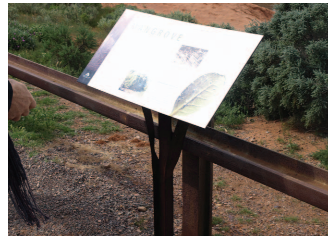
Rail reuse: Good example of re-use of former rail material.
