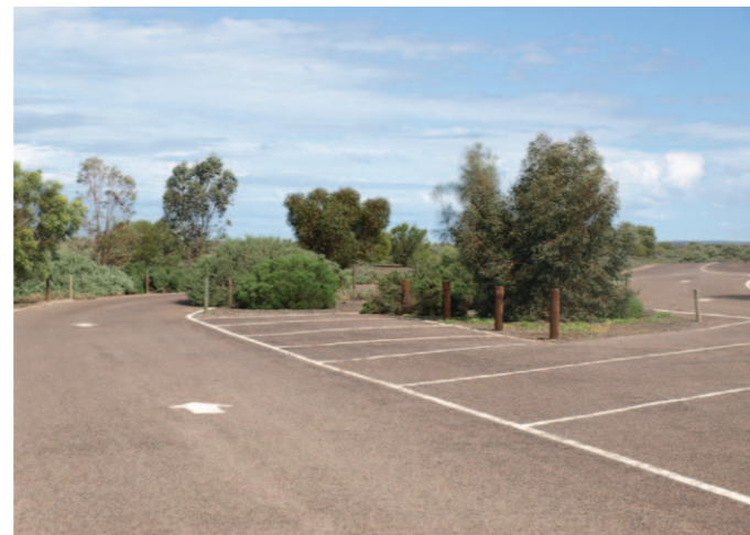
Carpark: Example of good carpark layout that is not 'over-engineered'. Use simple linework, appropriate Arid-Smart planting and minimal signage.
