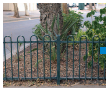
Existing: Painted 'pool' fence
